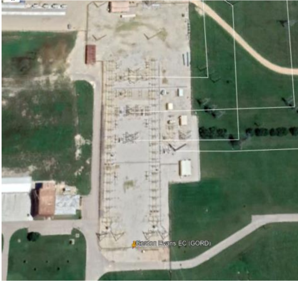
Figure 33 – Gordon Evans 138kV Substation
